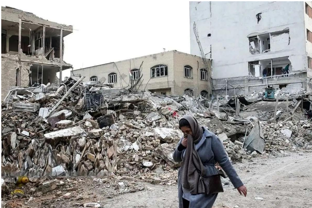
Figure 3. Residential buildings in Iran destroyed by airstrikes during the 40-day conflict. The Iranian Red Crescent Society recorded more than 125,600 civilian units damaged nationwide, including at least 1,246 completely destroyed — a scale of destruction approximately 15 times greater than the June 2025 Twelve-Day War.
