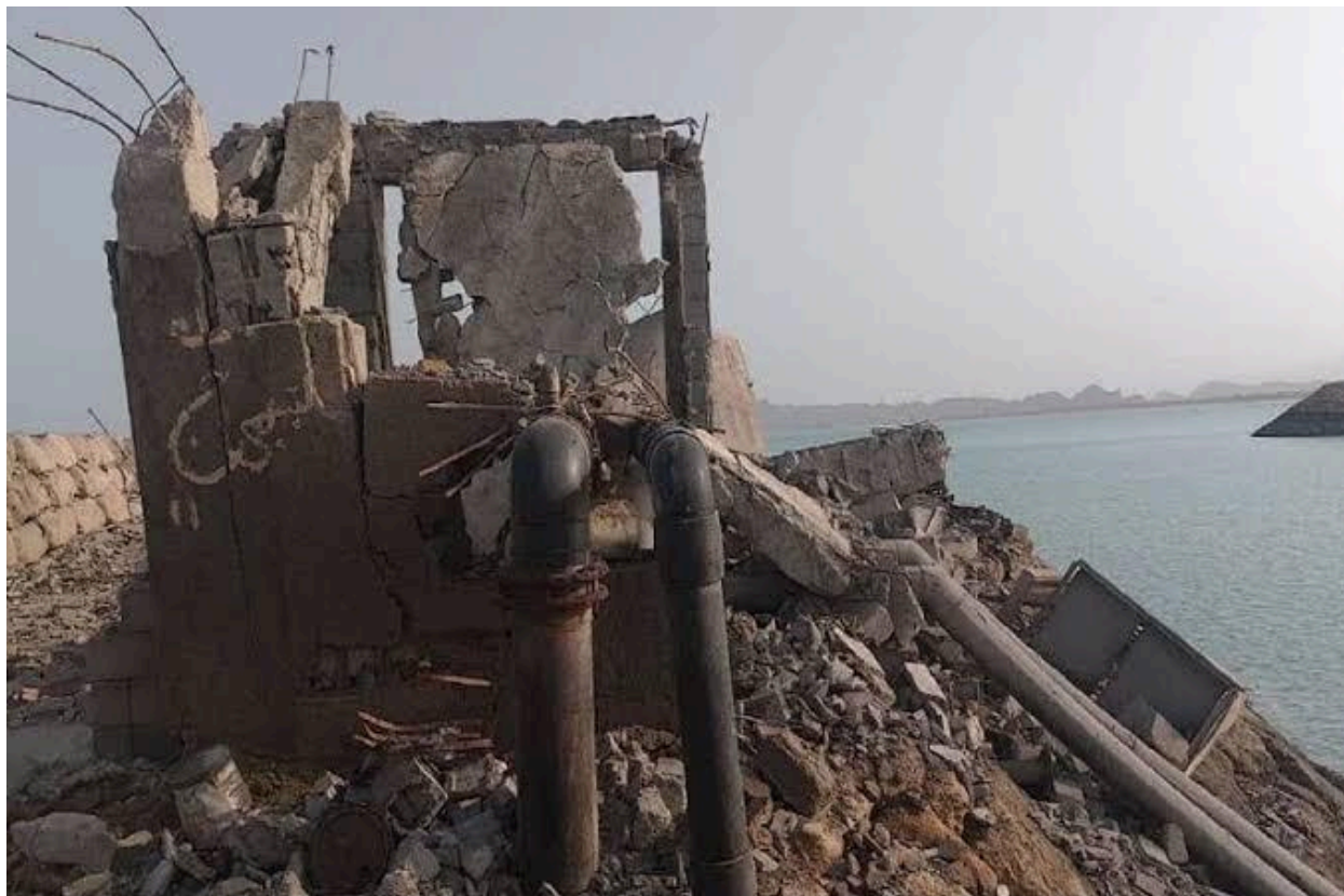
Figure 8. The Bonji desalination plant in western Jask county, Hormozgan, after the US strike of July 18, 2026. The seawater intake pumping station and electrical transformer were destroyed, cutting drinking water to 20 villages of some 10,000 people, until it was restored. Credit: IRNA.
