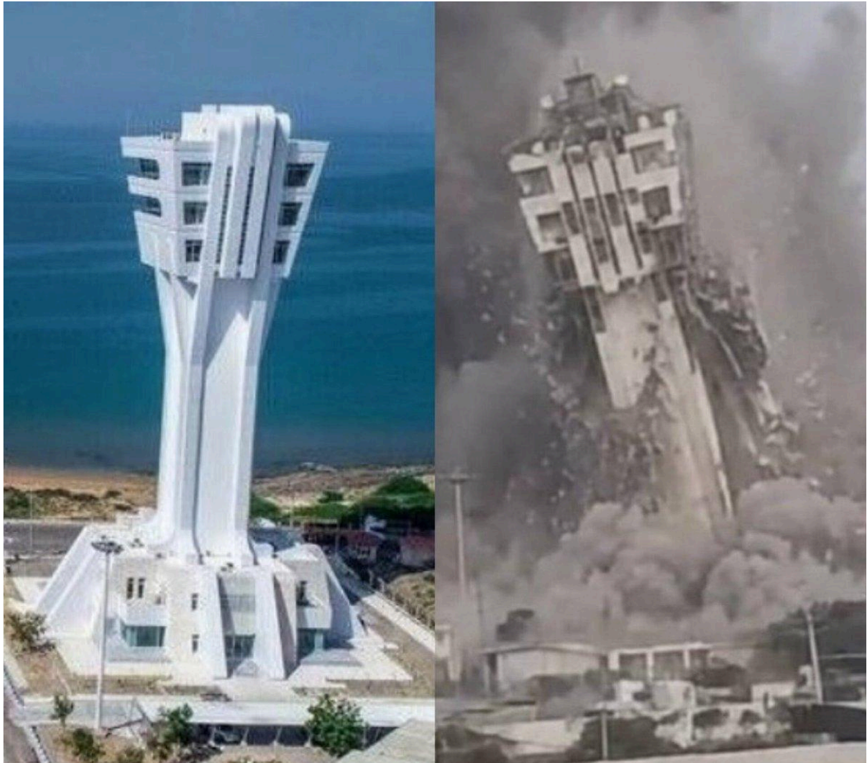
Figure 6. The marine traffic control tower at Chabahar port, destroyed in Phase II strikes alongside the Bushehr Meteorological Center and fishing infrastructure on Qeshm Island — facilities on which coastal shipping safety and fishing communities directly depend.
